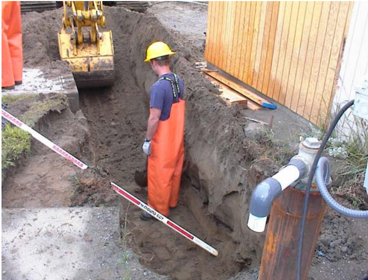
- Crew installing a new water main
