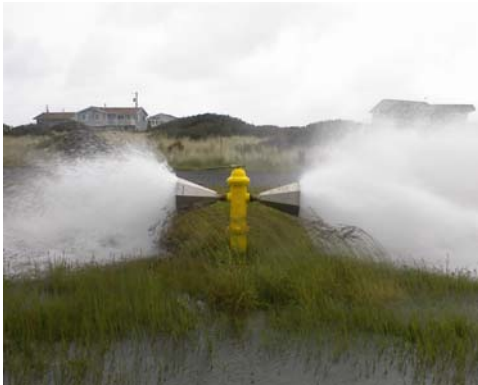
- Flushing a water main
